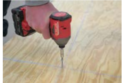
FIGURE 5: Attaching the plywood
