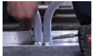
FIGURE 10: Bolting the railing
