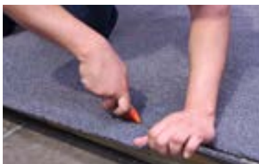
FIGURE 8: Trimming the carpet
