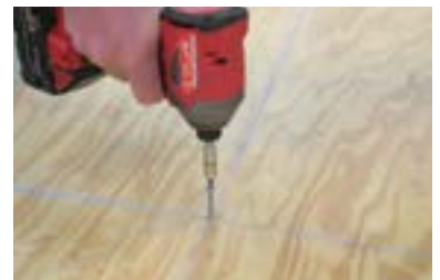
FIGURE 4: Attaching the plywood
