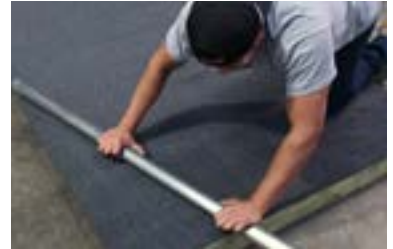
FIGURE 7: Rolling out the carpet
