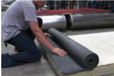
FIGURE 6: Laying the carpet
